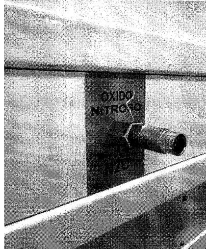
Figura 3 – ITEM 3: CONEXÃO MEDICINAL DE ÓXIDO NITROSO
